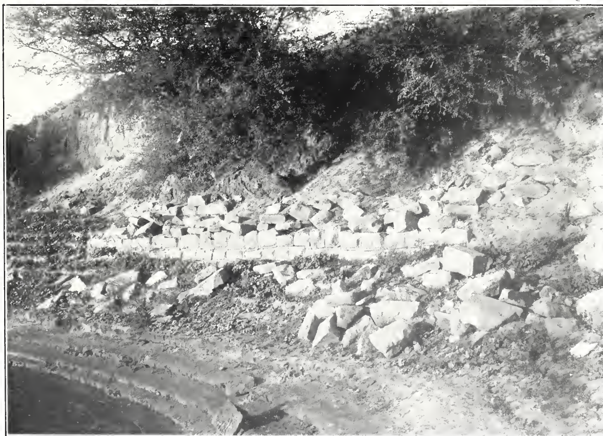
(b) Stone retaining wall on the river front at Shablul
